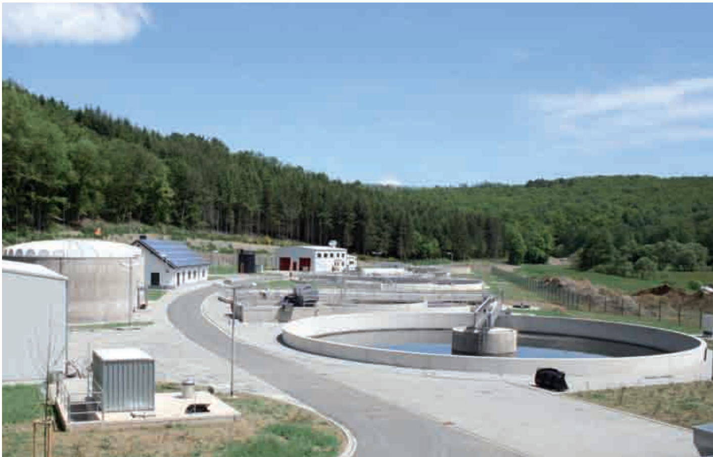
“Oberes Kyrbachtal” group sewage-treatment plant, ready for operation
