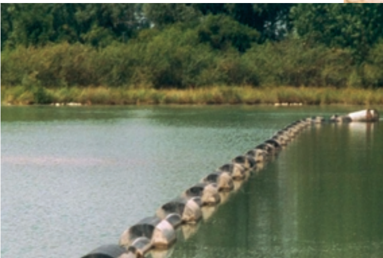
Outlet pipe to the centre of the lake for flushing out particles.
