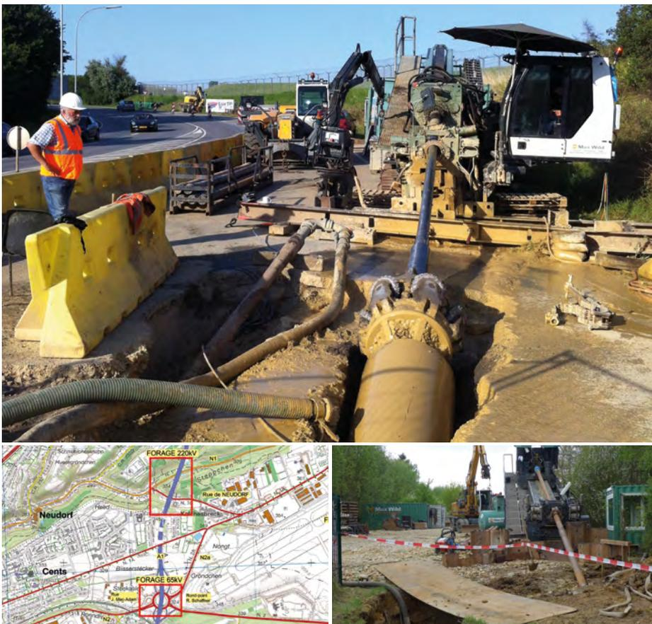
Top: destination pit with jetting tool – product pipe emerging in the destination pit with an attached hole opener; bottom left: the squares mark the locations of wash-boring operations; bottom right: the HDD method is performed by Max Wild, Berkheim, using a silenced 250 t wash-boring rig
