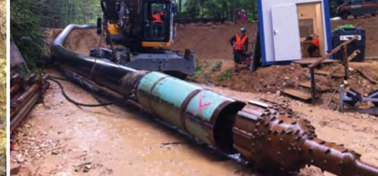
From left to right: connecting the pipe trains by heated-tool butt welding; SIMONA® PE 100 RC-Line Pipe with PE 100 empty conduits inside; welded pipe train for insertion into the starting pit with barrel reamer to widen and pre-ream the bored section
